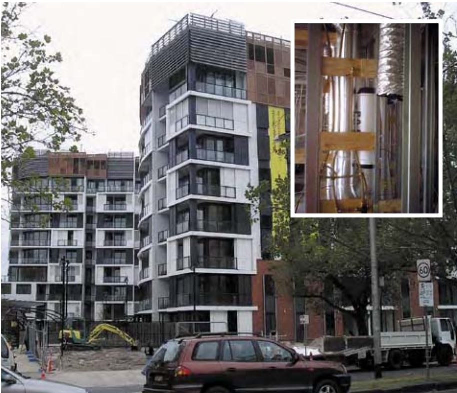
The new developments at the Chevron complex contain almost 300 apartments, yet the floor plans are inconsistent – a challenge for traditional plumbing design. Inset: The Studor P.A.P.A protects multi-level buildings from unwanted positive pressures, and can be installed in small spaces.
